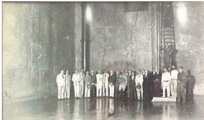
Inauguration of a completed reservoir constructed inside Waterworks East/West Tunnel
